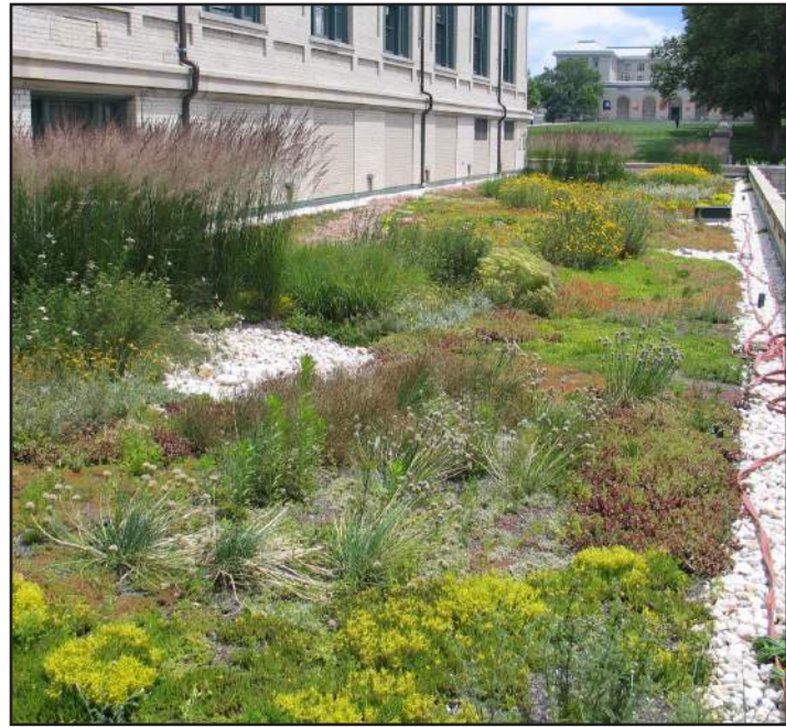
Figure 2.35 - Example of a semi-intensive green roof.
