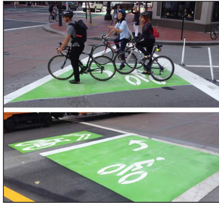
Figure 2.21 - bike boxes provide a safe place for bicycles to use an intersection
