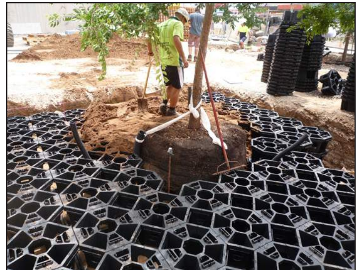
Figure 2.06 - The suspended pavement system involves a tree being planted on a grid over which pavement will be laid.
