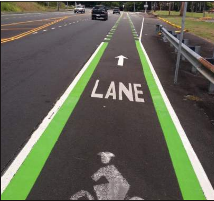
Figure 2.20 - Simple bike lane, using only paint to separate car and bicycle traffic
